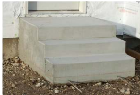
B Concrete steps
