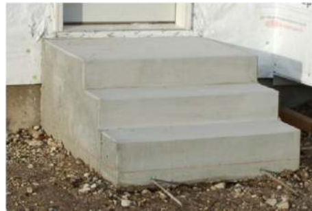
B Concrete steps
